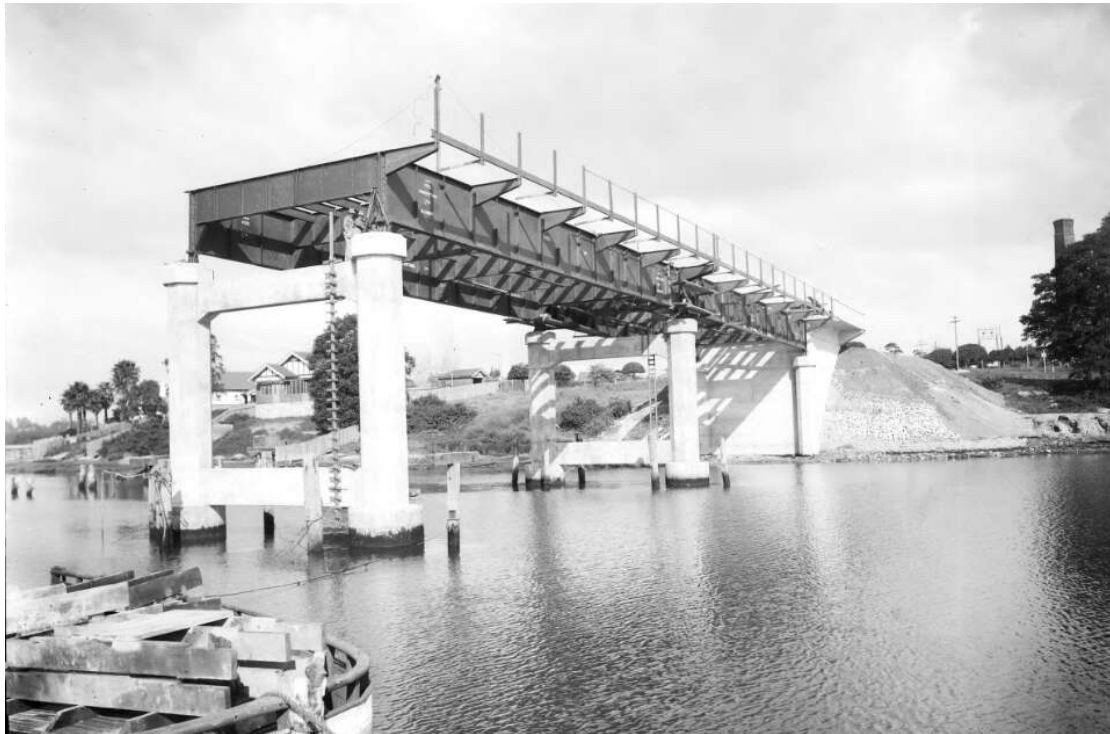
C1950s Initial Construction of the road bridge, showing the current Uhr's Point and abutments (Source: National Library of Australia)
